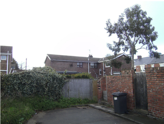
View of rear of property looking North
