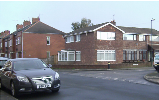
View of front of property looking South
